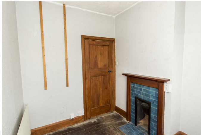
Single-glazed window to rear. Radiator.
