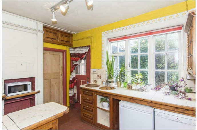
Window to rear. Fitted range of wall and floor mounted kitchen units. Space and plumbing for various appliances. Radiator.
