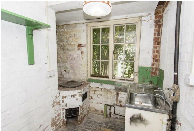
Utility 9'8" x 6'0" (2.95m x 1.83m)
