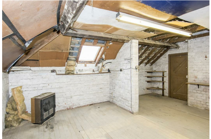
Double-glazed Velux skylight to rear. Window to front.
