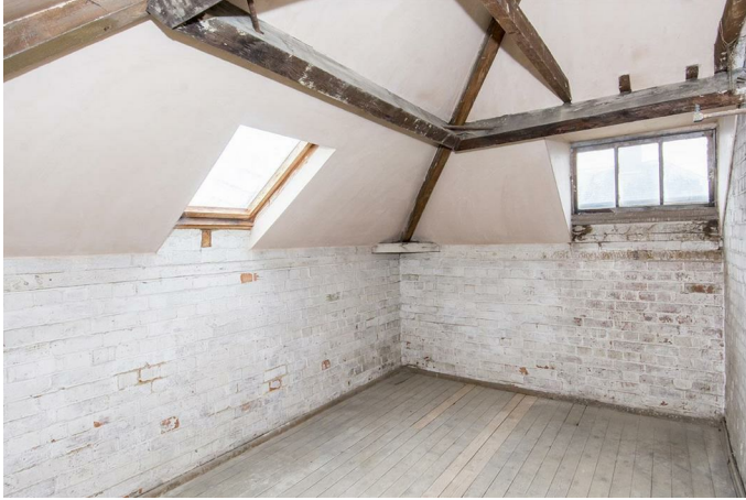
Timber door. Velux skylight to side. Window to front.
